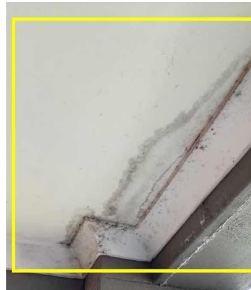
Clear evidence of leaks
