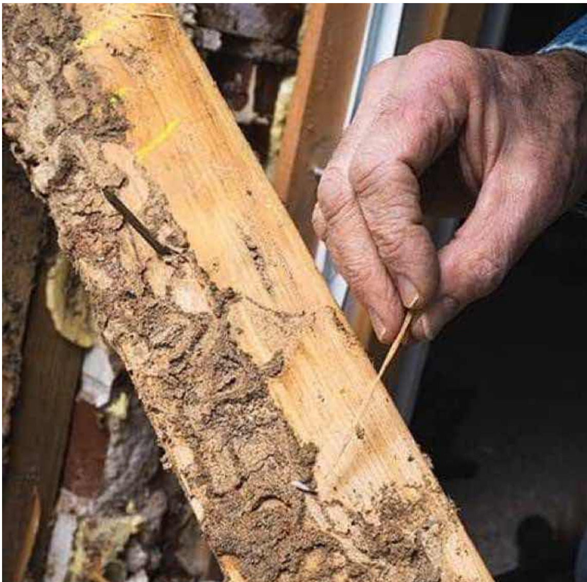
Roof framing timber
